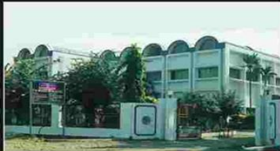
Manufacturing Plant II - Umbergaon, INDIA
